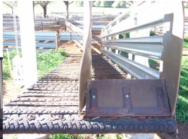
Picture 3: A ramp using old truck tyres across the floor to provide quiet grip. Photograph E Joshua.
