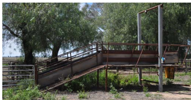
Picture 1: An adjustable ramp for a variety of sheep floats heights. NB there is a level entry to the float at this height and safety rails for the operator. Photograph by E Joshua.
